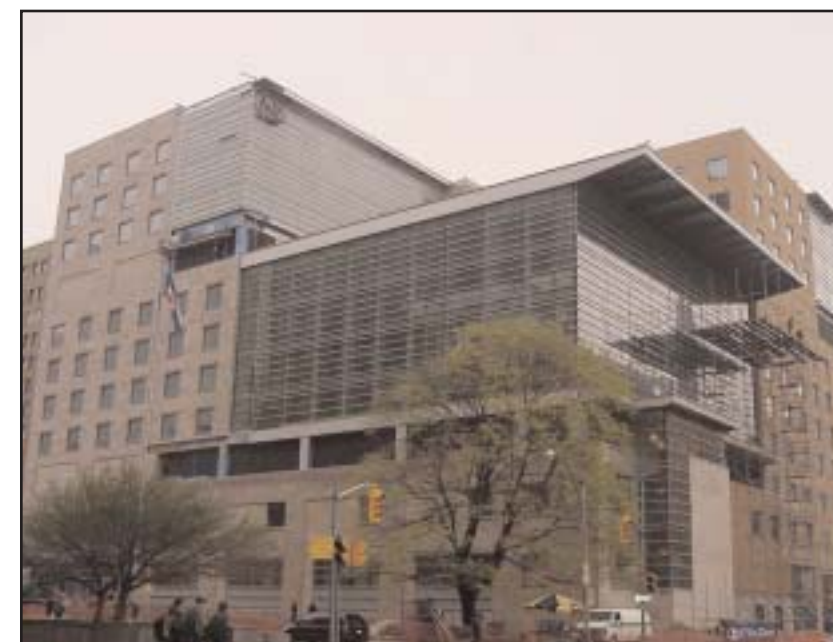
The Clinical Services Building at the corner of University Avenue and Gerrard Street
